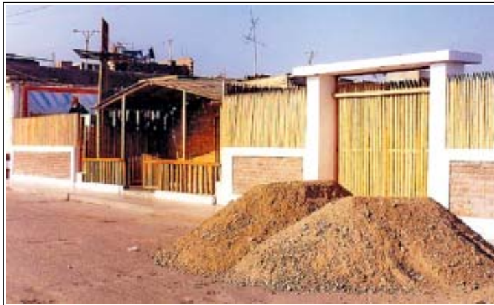
Construction work on the parish grounds of San Francisco de Asis.
